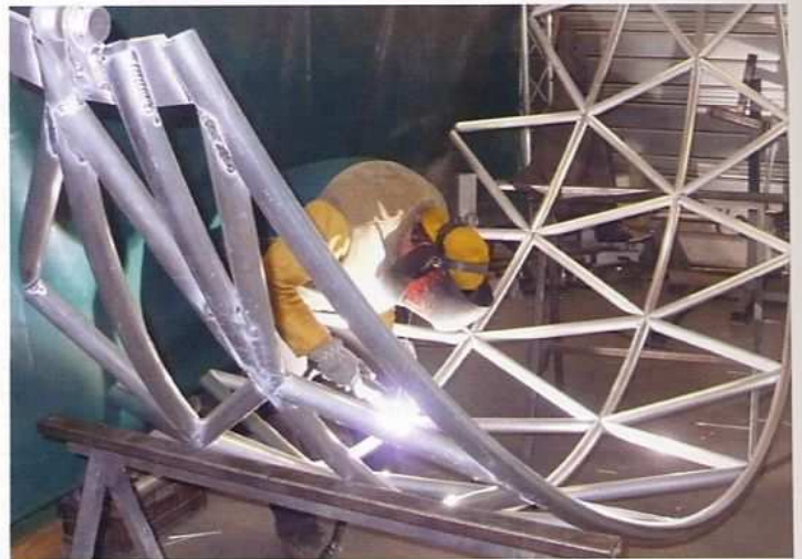
A section of the aluminium sphere in manufacture in FL Structures' soldering and welding department.
