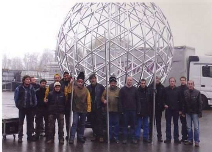
The FL Structures team show the completed sphere before Sky Light added their touch of colour.
