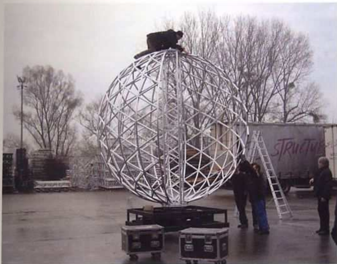
The first test of rigging the sphere in FL Structures' yard.
