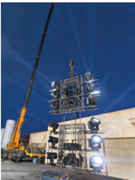
Dual truss frame mounted with 12 Syncrolite SXB-5/2s ready for flying.
